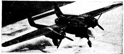
FIG. 9.11.-P-61 airplane with nose radome.
