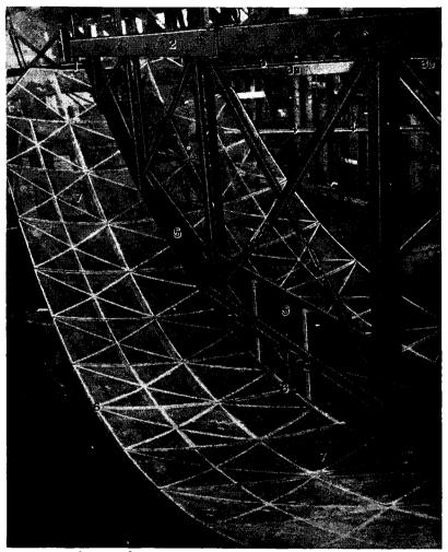
FIG. 24.—Reflector and template. (Courtesy of Walsh Construction Company.) 1. Template rotary truck. 2. Top chord of template truss. 3. Track. 3a. Track support. 4. Walkway. 5. Template. 6. Center support. 7. Reflector.
